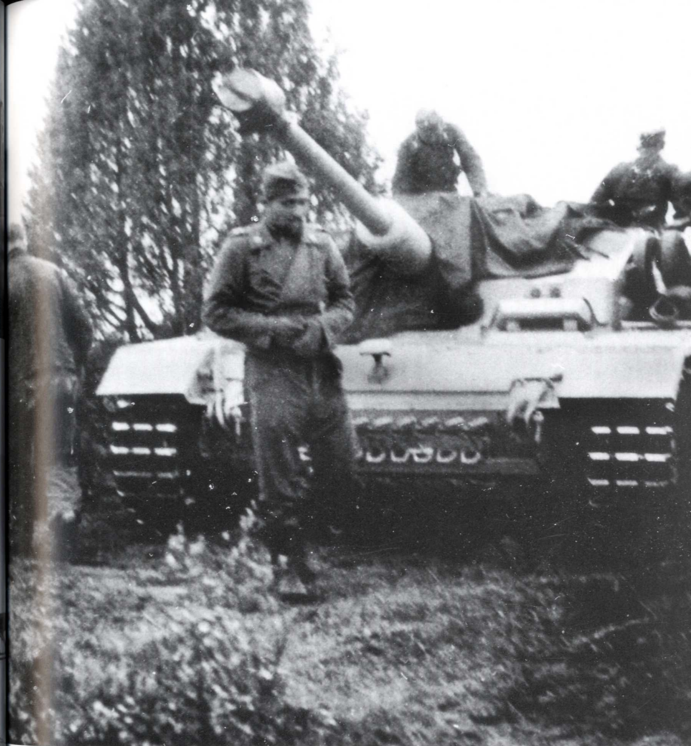
The crew of a Ausf.F have halted in a field during a pause in operations somewhere on the Eastern Front. Note the tarpaulin fitted around the welded gun mantle and the casemate roof. This was done in order to keep the assault gun dry from the elements.
