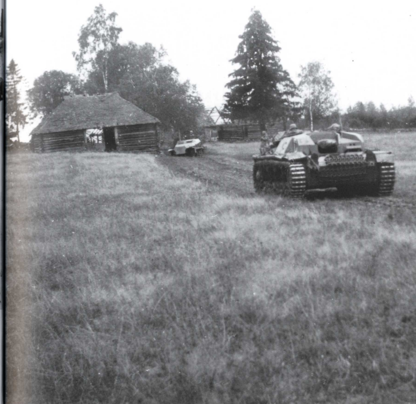
An Ausf.B variant advances through a field. This apparent experienced crew has used spare track links to create additional armored protection to the front of the vehicle's superstructure. Behind the StuG is an Sd.Kfz.252 which was a light armored ammunition transporter for the Sturmgeschütz units.
