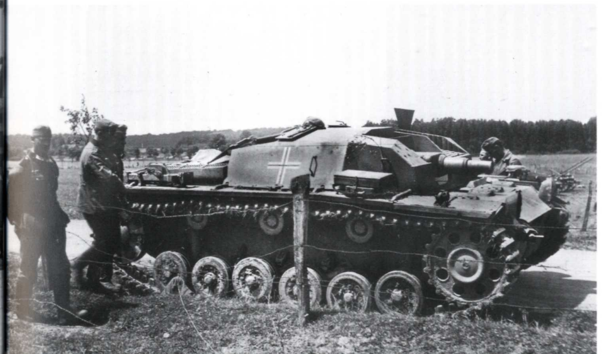
Two photographs taken in sequence showing a StuG.III has halted beside a road. This Ausf.B variant displays quite nicely its wider 40cm tracks, and by the appearance of mud and grass has undergone some cross-country driving. Note the Notek driving head-lamps mounted on the front of the vehicle. These lights could also be blacked-out.
