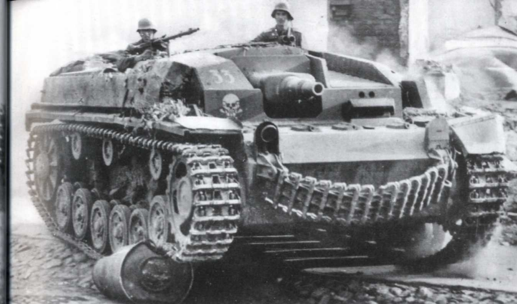
An Ausf. B variant belonging to the Sturmartillerie-Abteilung 192 moves through a town during an urbanized contact in the summer of 1941. Note the track links attached to the front superstructure of the vehicle for additional armoured protection. By the time the Germans attacked Russia the Sturmgeschütz battery strength increased to nine guns.
