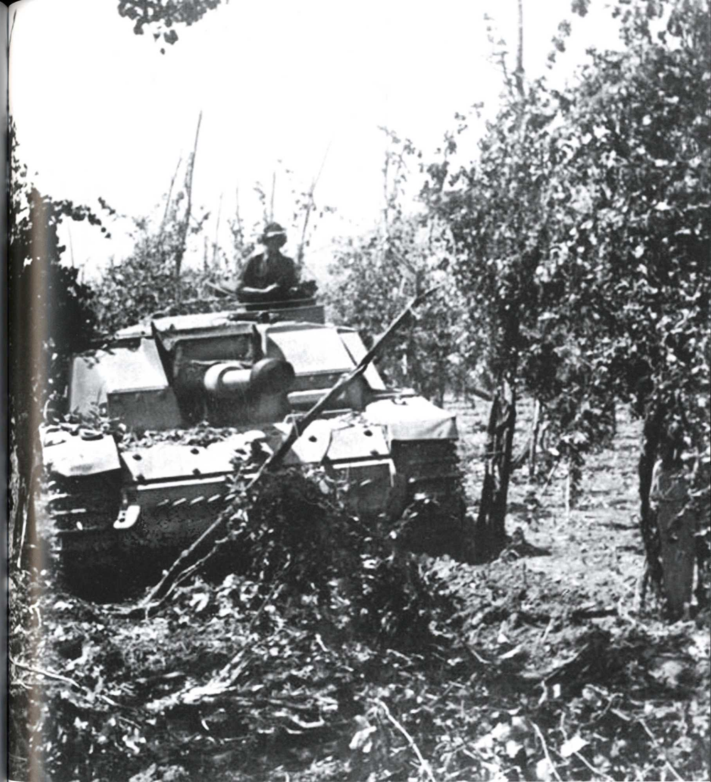
A StuG.III.Ausf.G has halted in what appears to be a orchard during operations in northern Italy in 1944. Note the distinctive commander's cupola. Also of interest is the tarpaulin protecting the mantle of the gun.
