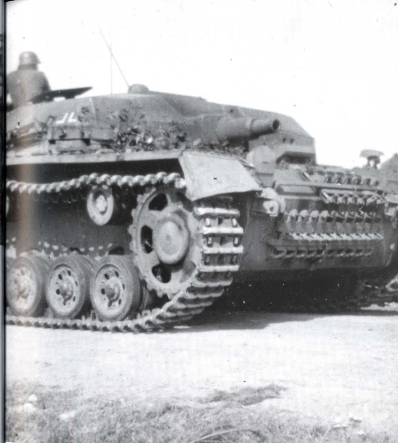
An early variant StuG moves along a road. The vehicle has received two track links attached to the front of the superstructure in a drastic attempt to mitigate against penetration of the thin armour by Russian infantry anti-tank rifles.
