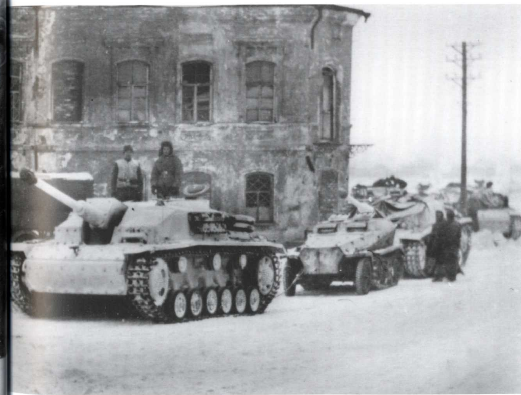
A new whitewashed StuG.III Ausf.G variant in a field. This was the final variant to be manufactured, and it came off the production line in 1943, and was rushed straight into service. The Ausf.G was armed with an MG34 for local defence and featured periscope to give the commander some protection as he surveyed the local terrain.
