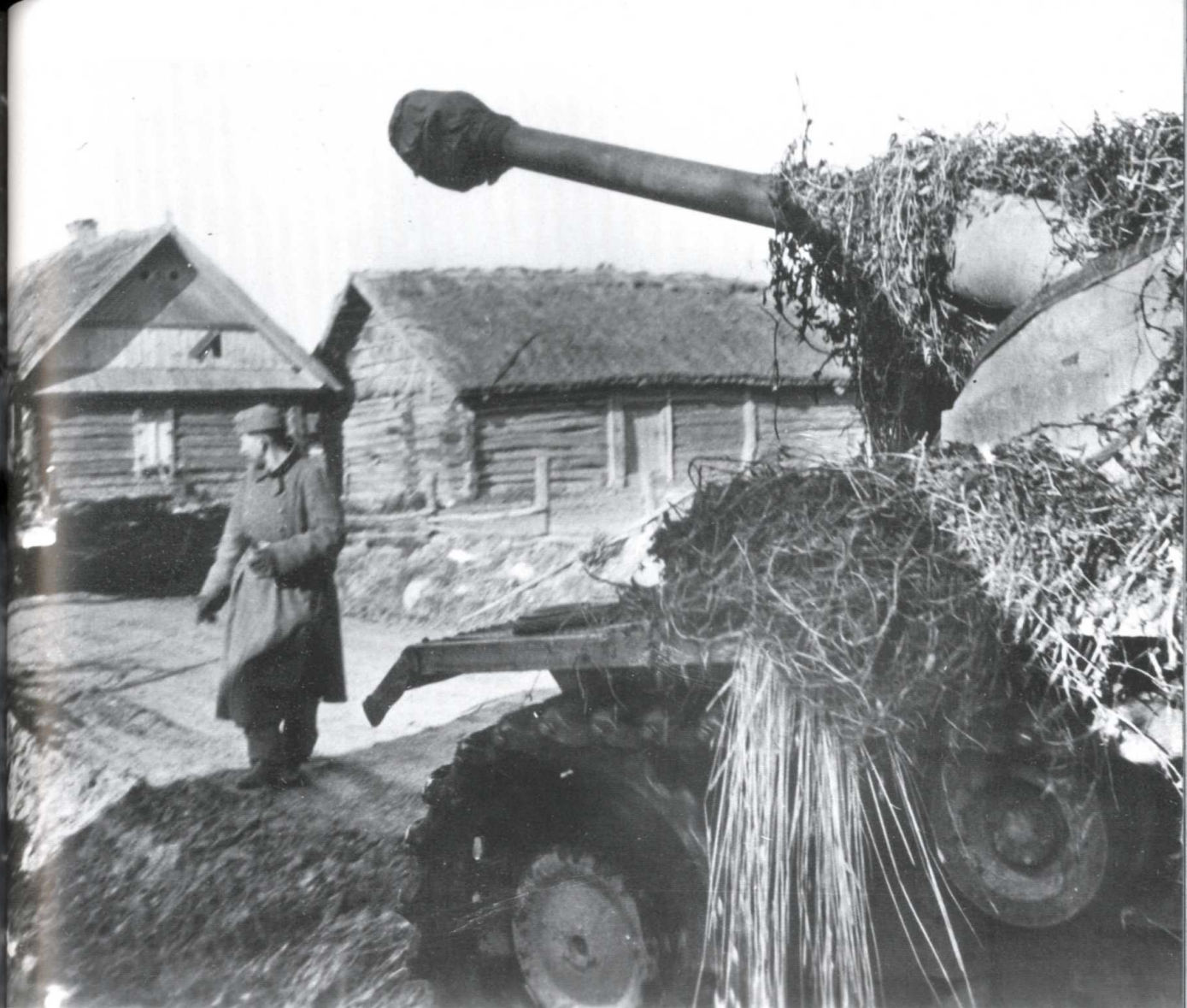
An interesting photograph showing an Ausf.G variant with what appears to be a concrete-reinforced frontal superstructure. Note how the crew has camouflaged part of the hull and bottom part of the 7.5cm StuK40 L/48 gun barrel.
